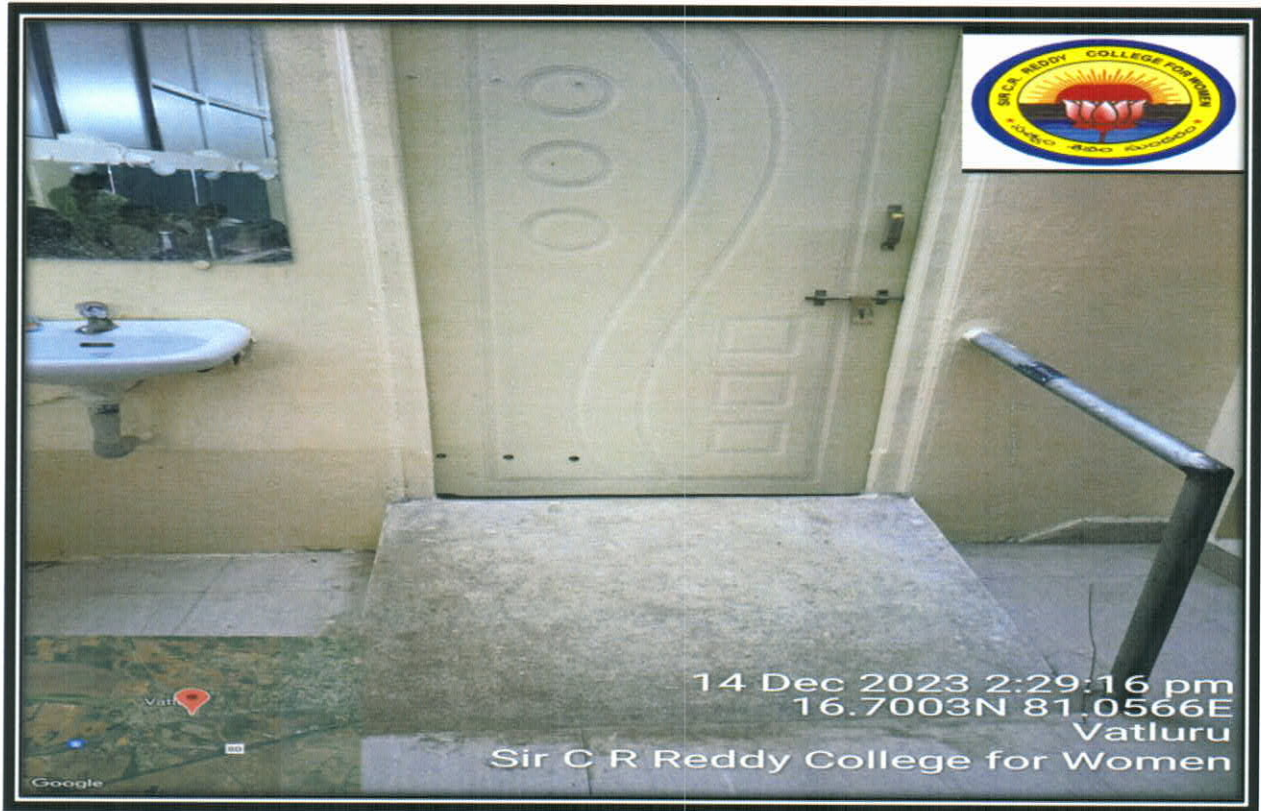
Ramp for Divyangan at Rest Room
