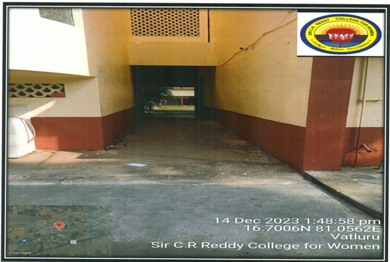
Ramp for Divyanggan at Degree Block
