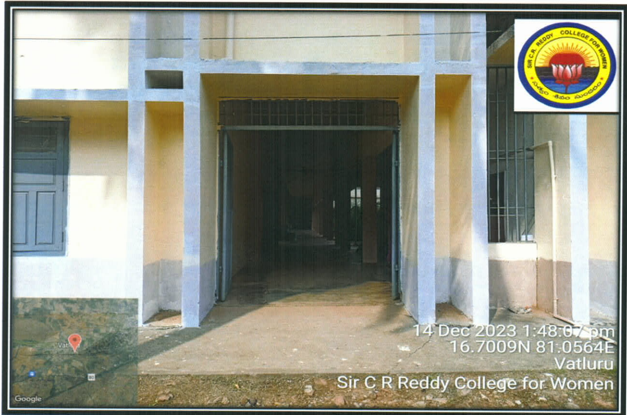
Ramp for Divyangnan at PG Block
